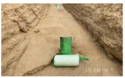
type of erosion control mat. The PAM is then hydrated either by humidity, wet soil conditions, or by manually wetting the material with a water hose. Once wetted, the material becomes a sticky gel-like substance that will gradually dissolve with the storm water flow in the swale. The swale should flow to a sediment basin where the floc can settle out.
